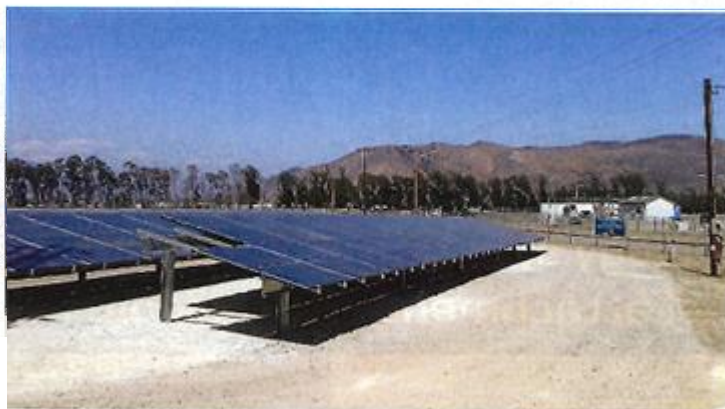
REC Solar developed this 1 MW PV installation for a jail facility in Ventura County, Calif. Photo courtesy of REC Solar
