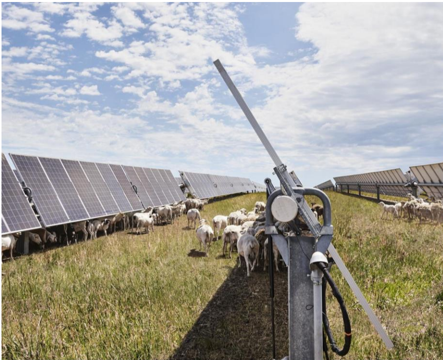
Example of solar panel rotation at North Star Solar, MN
