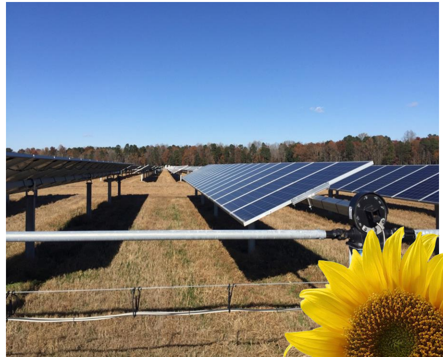
Example of solar panel rotation at Amazon Solar, VA
