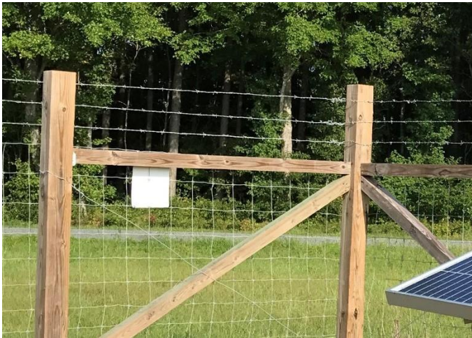
Fence at Elizabethtown College Solar, PA
