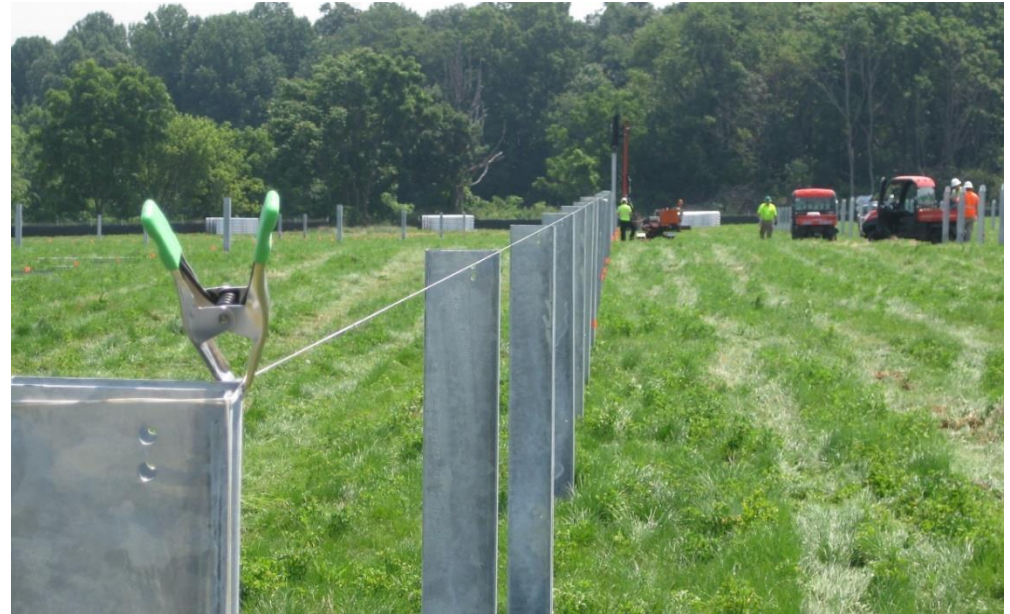
Example of post installation during construction of Keystone Solar, PA
