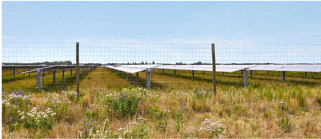
Example of agricultural style fencing at North Star Solar, MN
