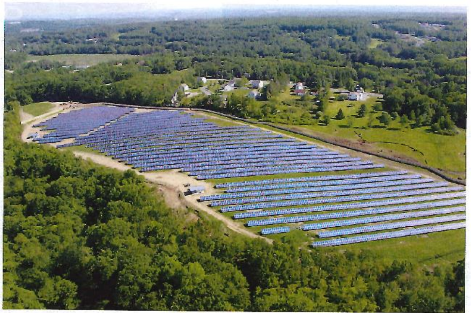
One of two 1 MW solar projects Community Energy developed for the Town of Sterling, Mass. Photo courtesy of Community Energy
