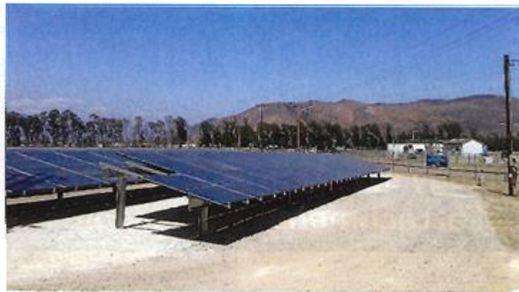
REC Solar developed this 1 MW PV installation for a jail facility in Ventura County, Calif. Photo courtesy of REC Solar
